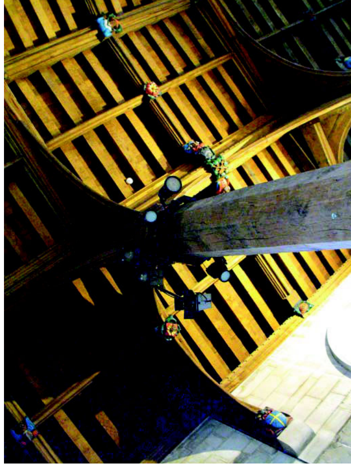
Interior timber frame structure of the Guild Hall
